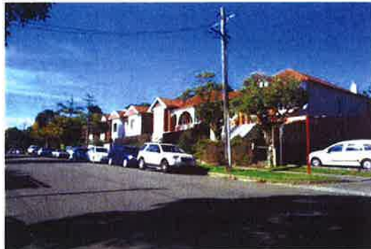
Photo 8: Photo of the neighbouring residential developments located along Atchison Street east of the site. Zig Zag Lane is located to the right. This portion of the road is proposed to be closed to vehicular traffic.
